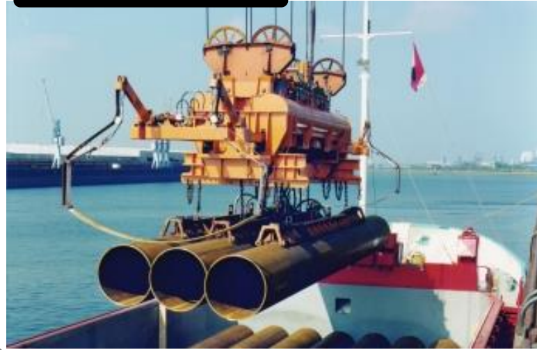
Handling of steel pipes
