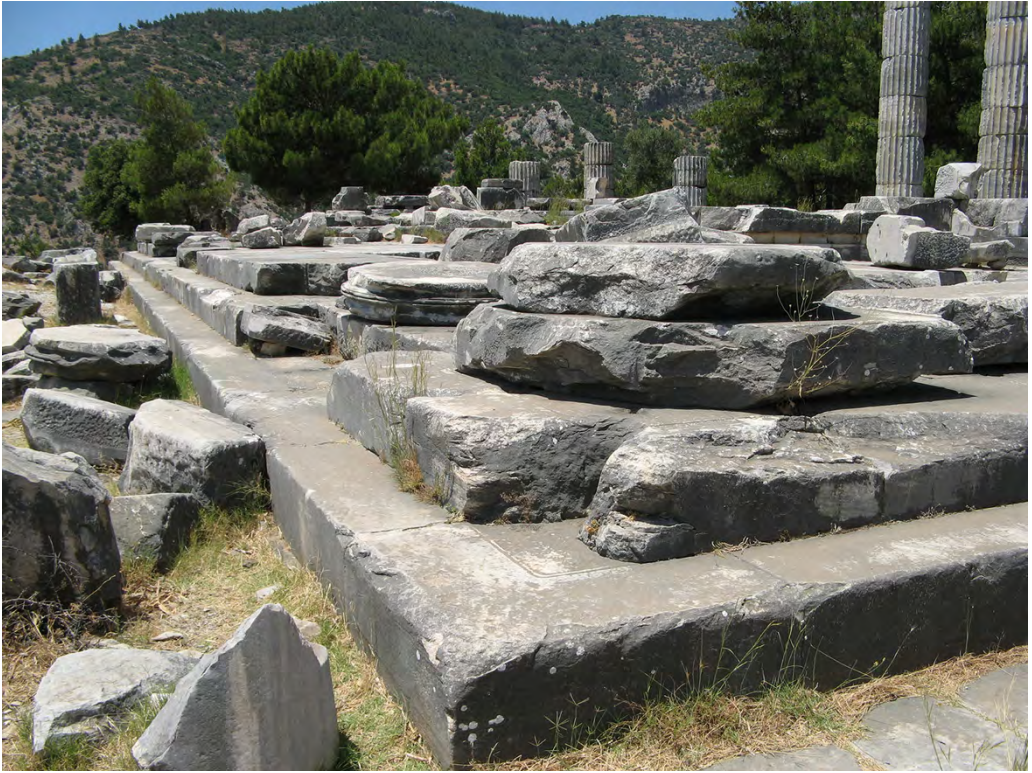
Figure 16.5 Temple of Athena Polias, Priene, northward view of stepped platform along west flank with visible curvature. Source: J. Senseney.
