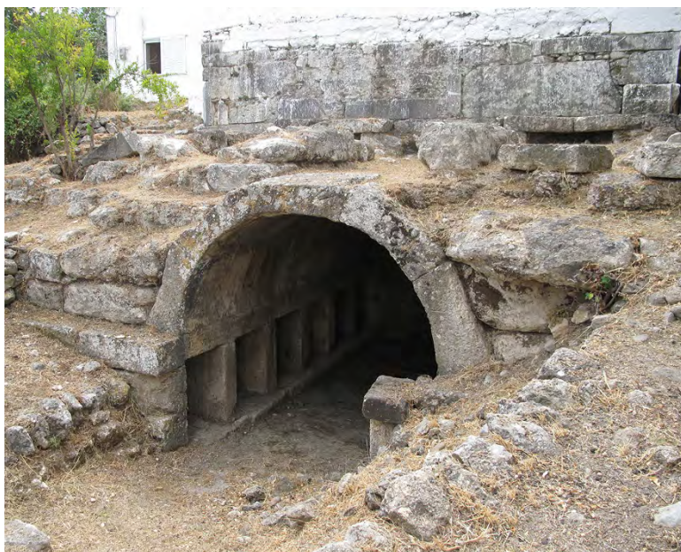
Figure 26.6 Vaulted crypt under the chamber tomb of Charmylos, Kos, third century BCE. Source: Olga Palagia.
