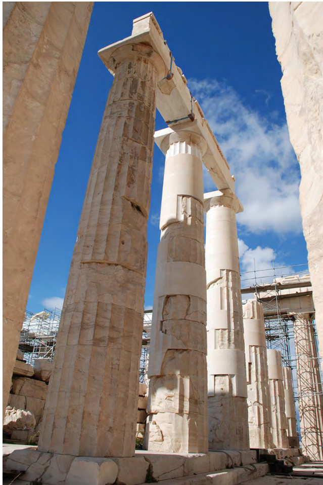
Figure 35.7 Implementation of Korres-Bouras' proposal for partial restoration of Pronaos 2004, view from southeast. Source: L. Lambrinou.
