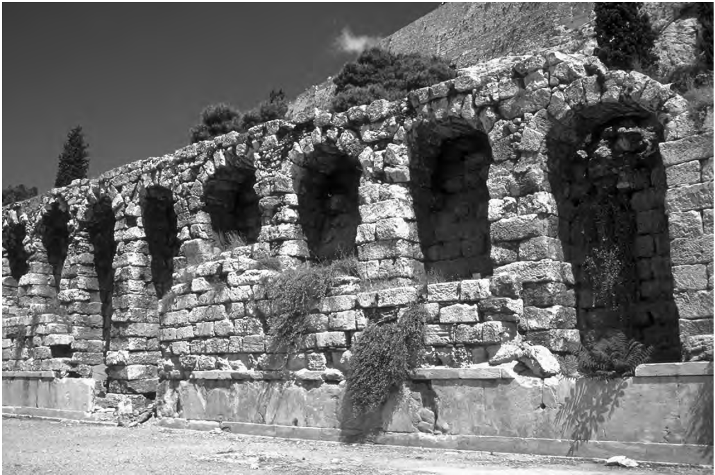
Figure 8.4 Stoa of Eumenes, Athens, view of arched buttresses. Source: N. Klein.
