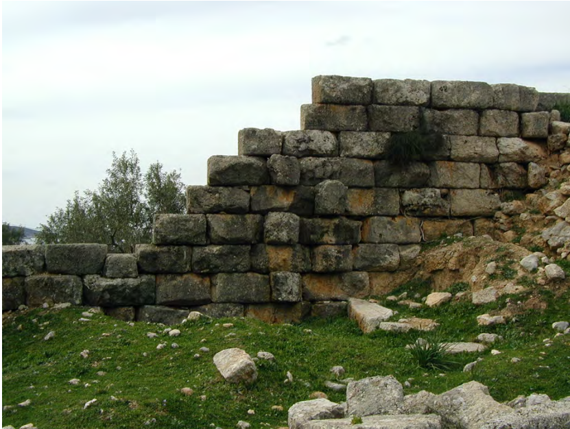
Figure 18.7 Chain wall masonry, Aigosthena. Source: S. Pope.
