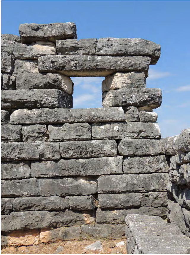
Figure 19.1 Orraon, andron, House A, stone construction and window. Source: B. Tsakirgis.
