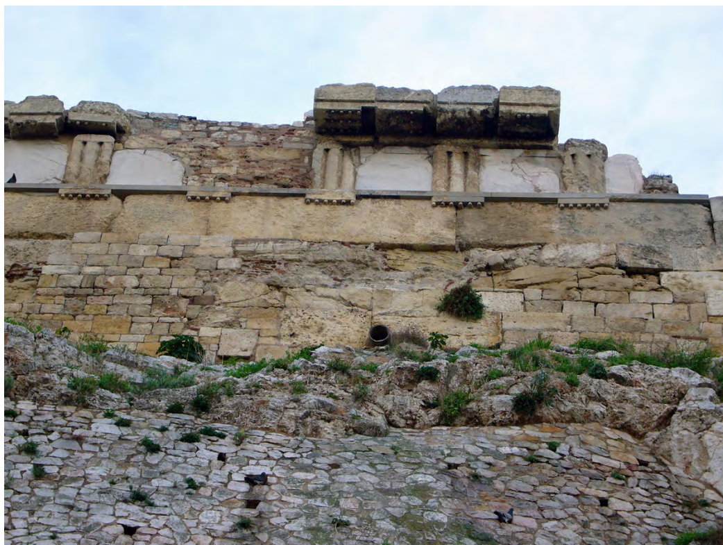
Figure 11.2 Acropolis, detail of north wall, with reused blocks from the Temple of Athena Polias. Source: M.M. Miles.
