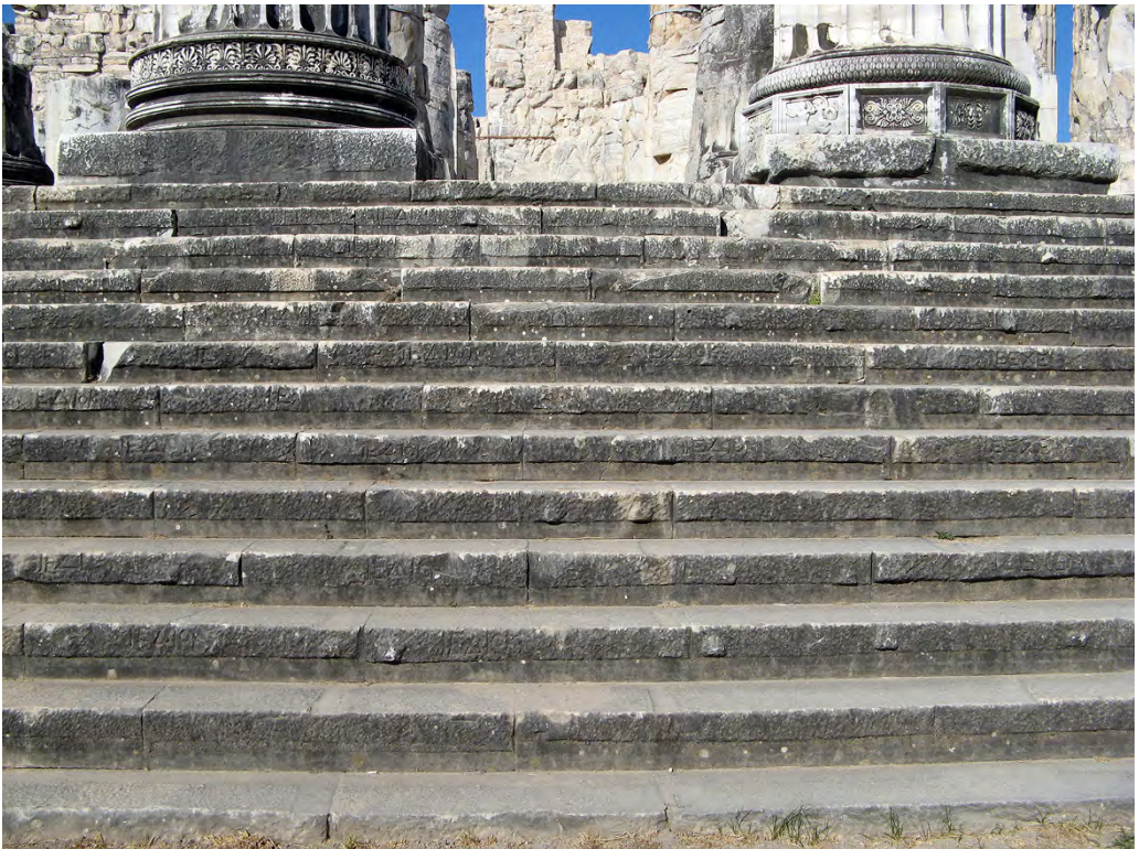
Figure 5.4 Sanctuary of Apollo, Didyma, view of frontal stairway ascending to stylobate, featuring panel-strips as found in the masonry of earlier Ionian temples as well as Lydian buildings. Source: J. Senseney.
