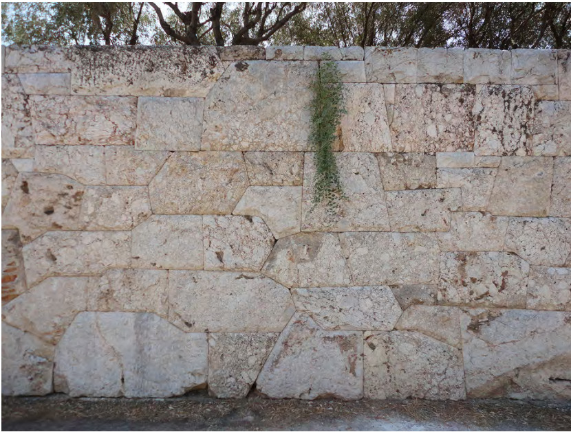
Figure 18.3 Polygonal masonry, Athenian Kerameikos. Source: S. Pope.
