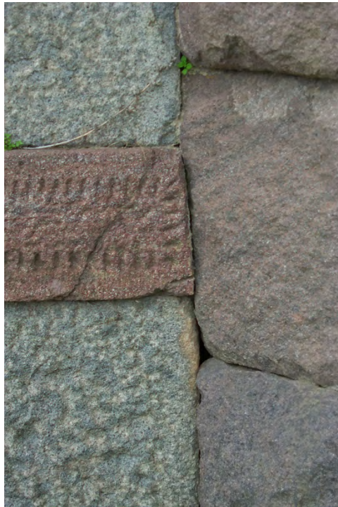
Figure 18.6 Chisel face finish on ashlar string course, Larisa. Source: S. Pope.
