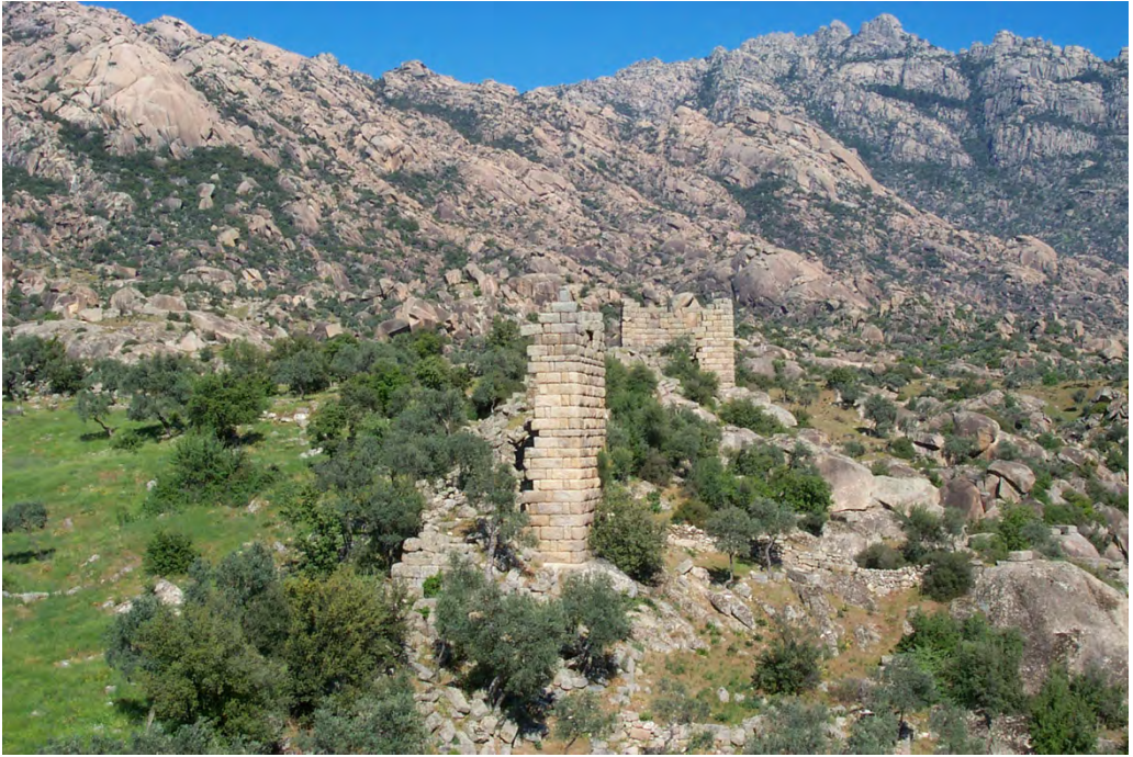
Figure 18.11 View of walls and tower, Herakleia-by-Latmos. Source: S. Pope.
