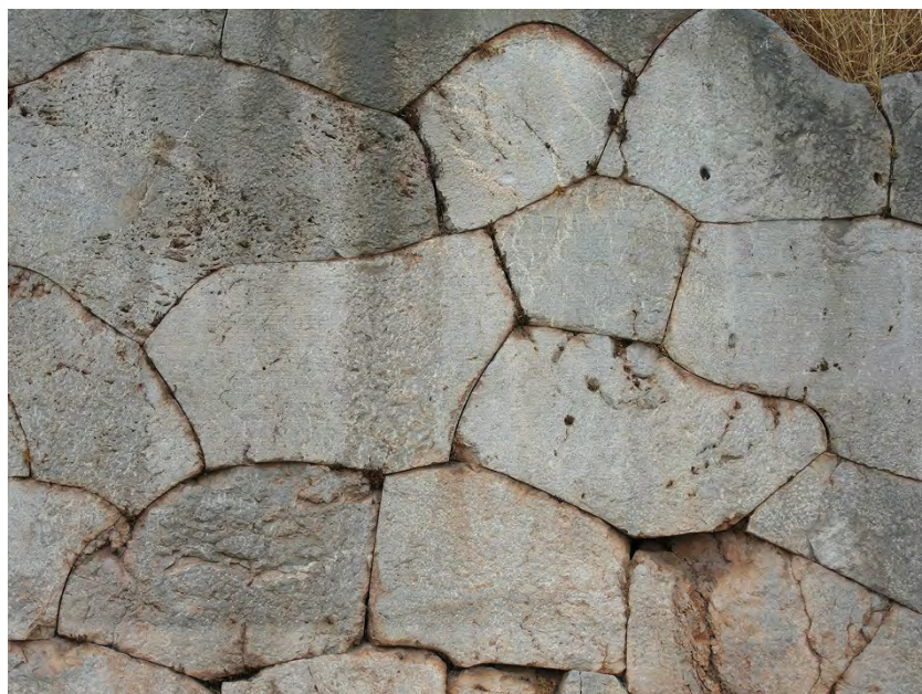
Figure 18.5 Curvilinear polygonal masonry from temple retaining wall, Delphi. Source: S. Pope.
