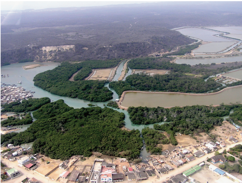
FIG. 16.47 Aerial photo showing patches of mangrove forest and excavated shrimp farms in Palmar, Ecuador. (Photograph by Windsor Aguirre)
