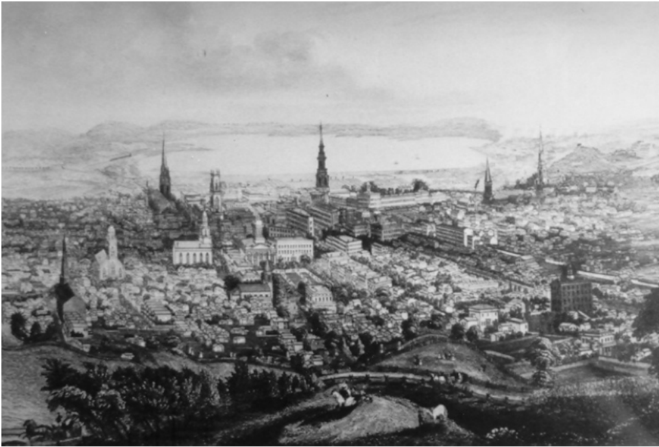
Figure 14.1 Bird's eye view of Syracuse New York, circa 1852. The image provides reasonably accurate historical information on the built environment even as it presents an opinion about the city and burgeoning urbanism in the mid-nineteenth century.
