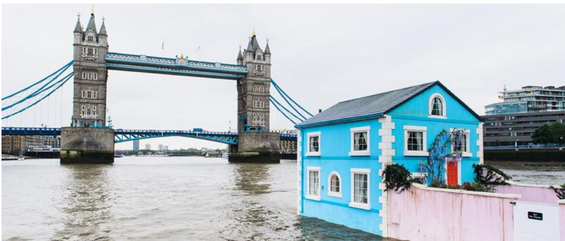
Figure 15: Accommodation - The Floating House, London
