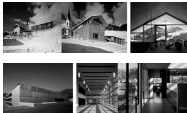
Fig. 3 (above) The primary and high school in Blons; (under) The infant-school in Egg.
