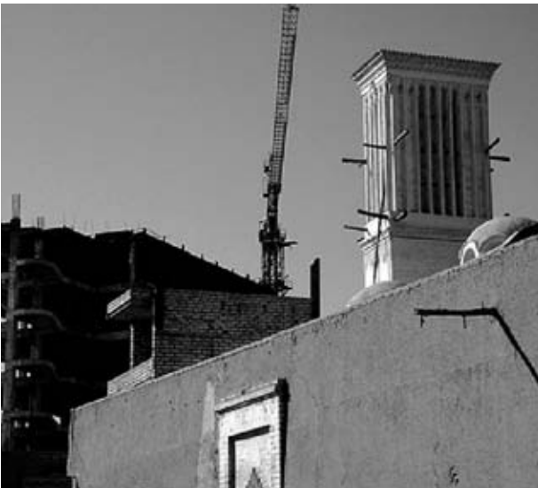
Fig. 6 New construction, Yazd http://www.mehrnews.com
