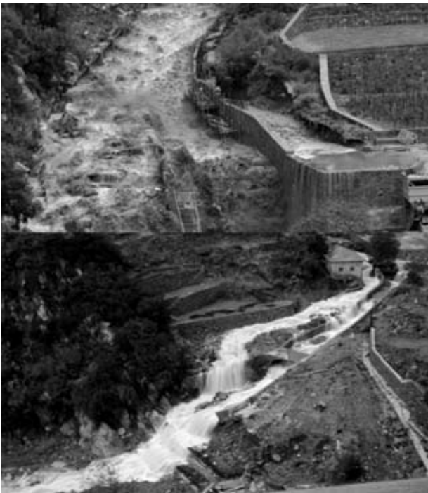
Fig 3.8 Characteristic views of a flood disaster in the stream Aeropotamos, Holy Mount Athos Dionysiou. Views of restoration works of the settlement system of the stream Aeropotamos (Pavlidis et al., 2012).
