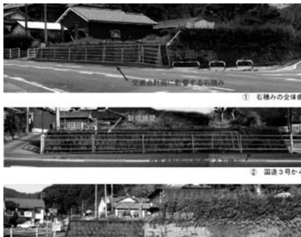
Fig. 6 Relation of new retaining wall (red) and the stone wall to be removed.
