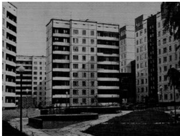
Fig. 1. Residential courtyard of Mezciems, Riga in the second half of the 20th century (Страутманис et al 1987).
