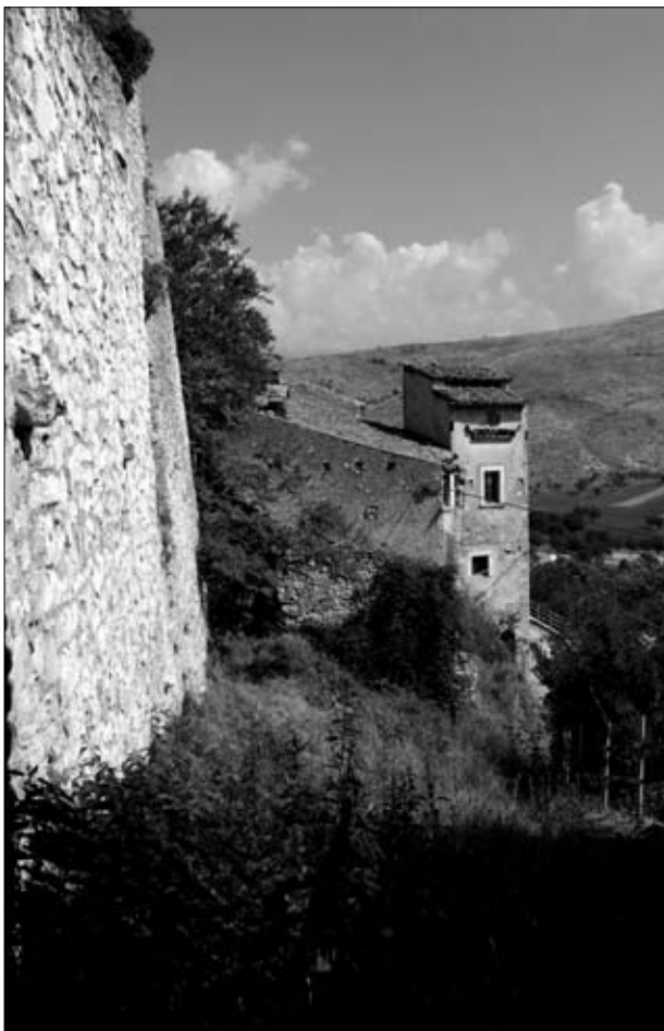
Fig. 2. Navelli (L'Aquila): building aggregates.
