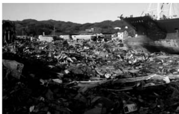
Fig. 1. (above) Near the port area
