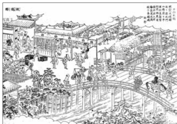
Fig. 6 Animated “Machiniwa” at bridge end
