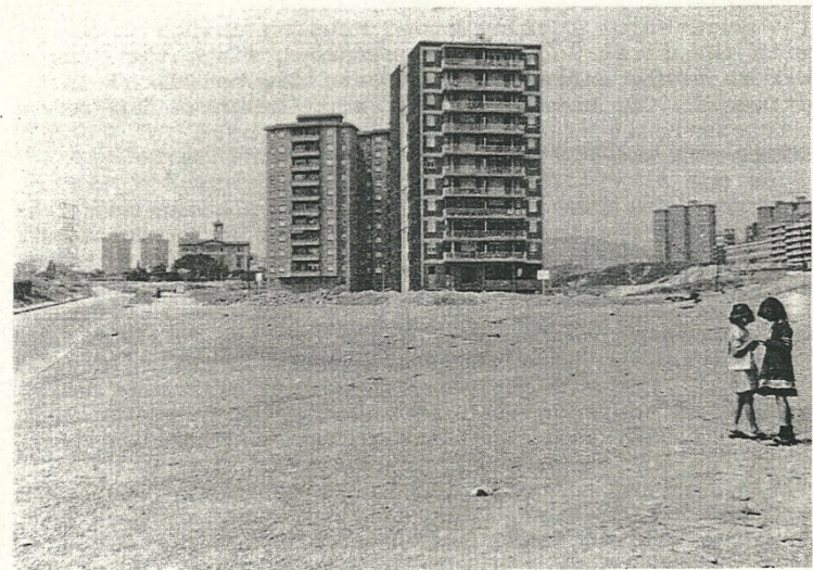
Figure 5.12 Can Serra, Hospitalet, Barcelona . Lack of local authority finances have often prevented the provision of service infrastructure contained in Local Plans for housing areas. Here, children play in an area in which a sports centre, public gardens, health centre and school should have been built. Photo: M.G. Wynn.
