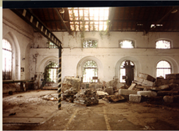
The Lamienni workshop before restoration
