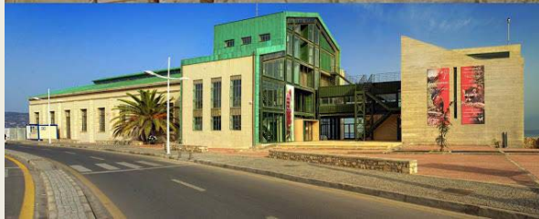
Old power station to natural history museum
