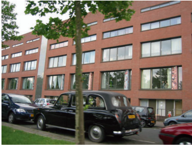
Figure 3 Bijlmermeer – new, owner-occupied building (photo by Susan S. Fainstein)
